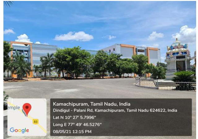
Fig. 10.2: View of all Buildings
